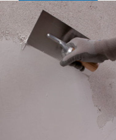
Spread on a first layer of Mape-Antique FC Ultrafine
