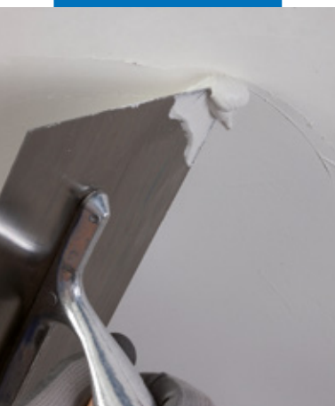
Smoothing over the product with a flat metal trowel
